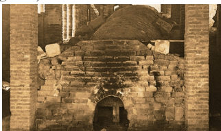
Traditional Chinese Dragon oven (龙窑 Long Yao), feeding mouth and filling method with electric porcelains (private collection)
